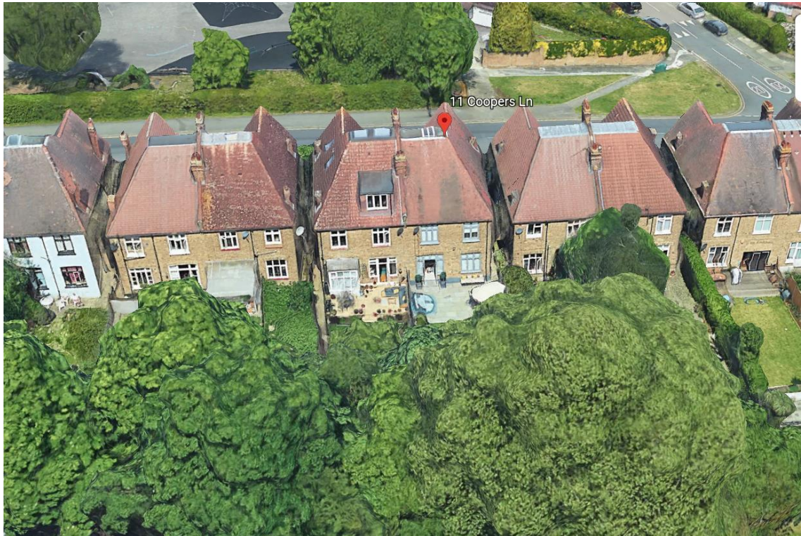
Figure 3. Aerial view to the Rear Elevation of No 11 Cooper's lane
